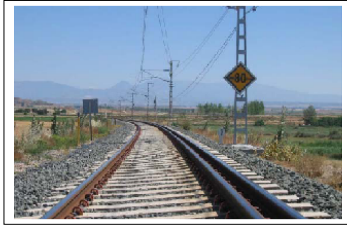
Figure 1. Three rails track (1668mm and 1435 mm)
