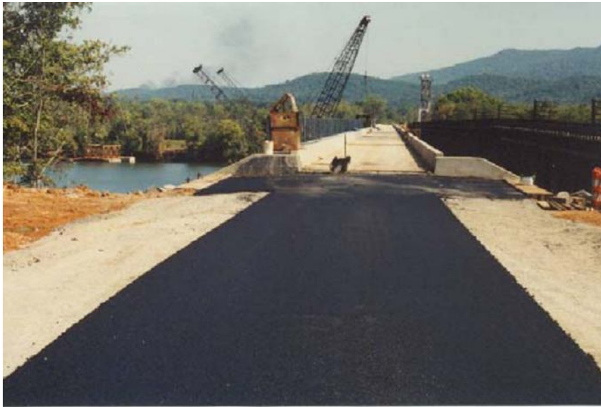
Figure 6. Bridgeport, Alabama bridge approach [9].
