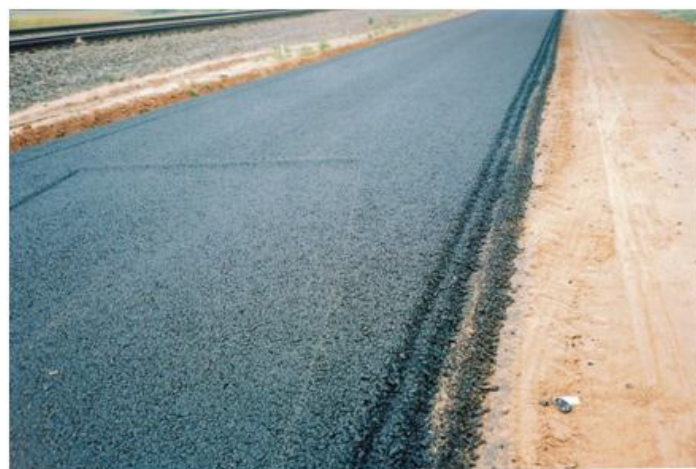
Figure 5. Aspect of asphalt trackbed for railway track [2].
