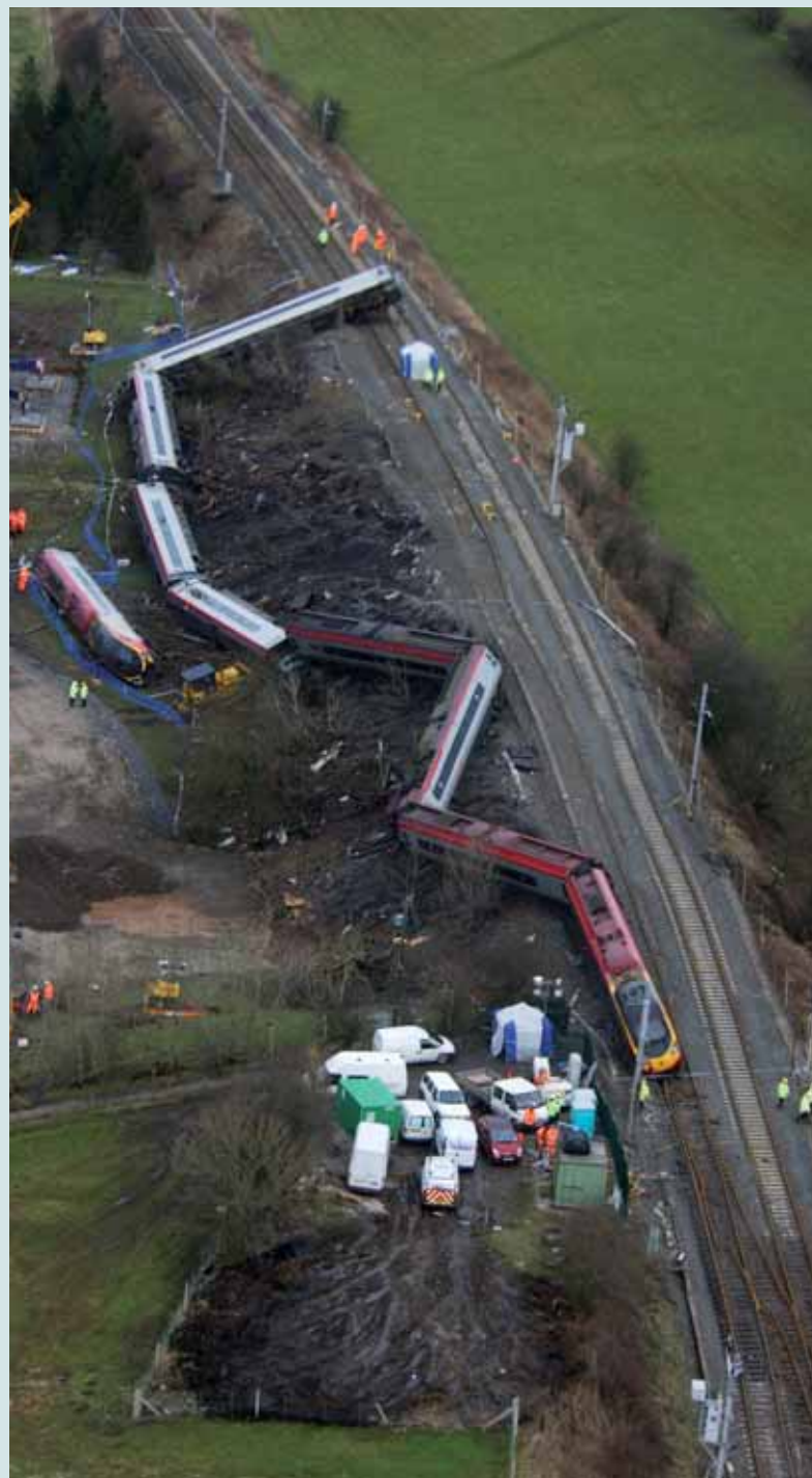
Figure 1 Passenger train derailment at Grayrigg in UK in February 2007 causing 1 passenger fatality and 5 serious injuries.
